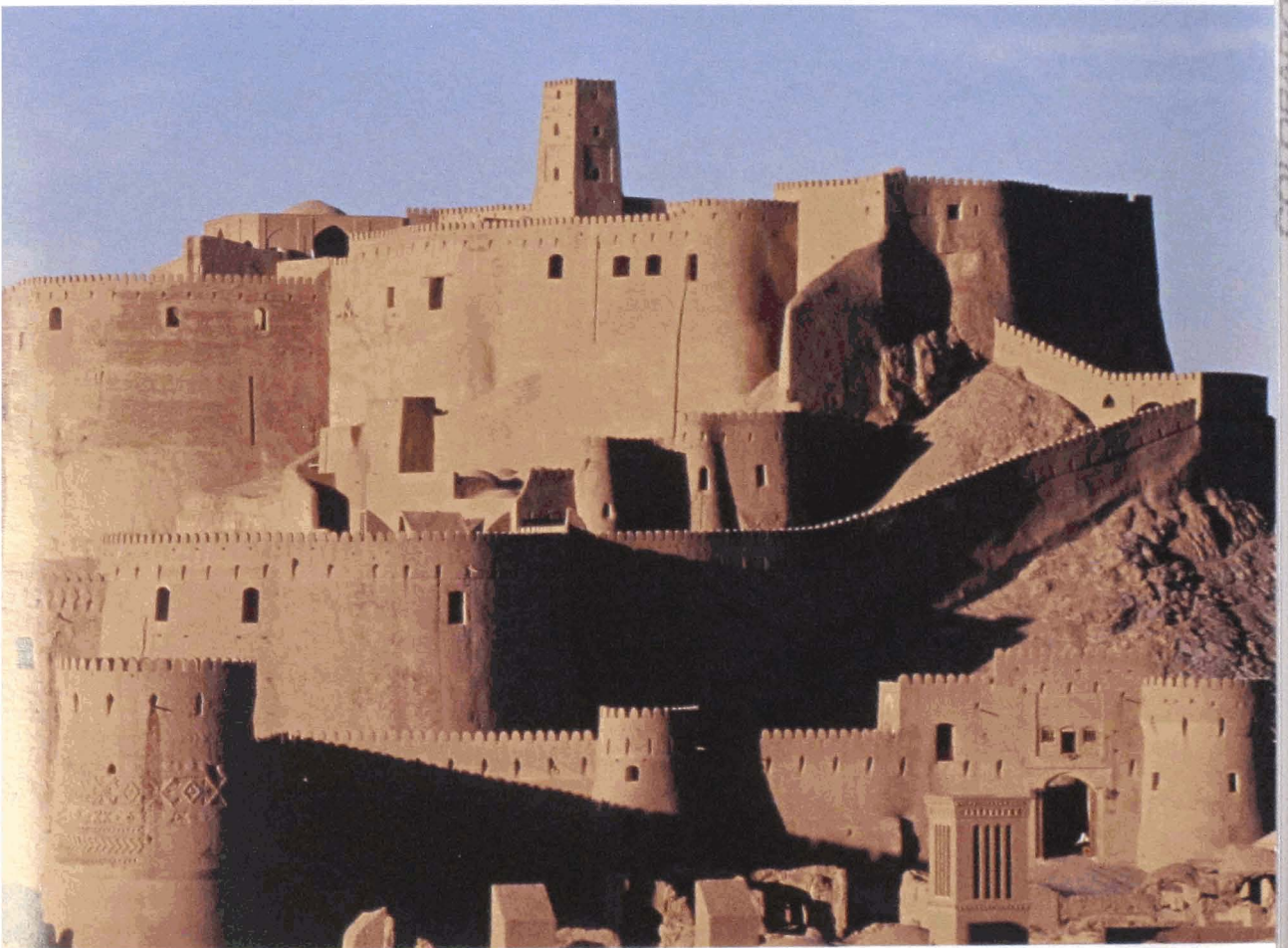
6 The citadel of Bam, Iran, destroyed by an earthquake in 2003
